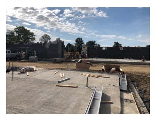
The exterior walls for the leisure pool and lazy river are all in place. Gutter installation along the outside edge of the pool is ongoing. Installation of the interior walls of the lazy river are scheduled for the week of August 3<sup>rd</sup>.
