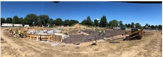
The excavation for the competition pool is done. Once the base has been installed, that too will be ready for the floor to be placed.
