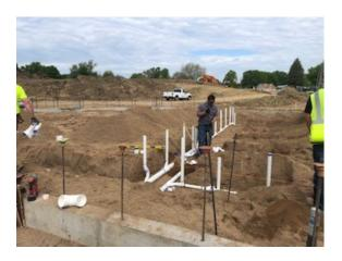
A layer of crushed rock is being placed in the lazy river area. This is on top of the sand that has already been installed. All of this is in preparation of the concrete placement.
