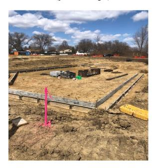
The hole for the lazy river and leisure pool has been dug and the drain tile has been installed. Backfill for the piping was in process.
