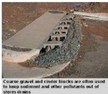
Diversion dikes can be used to contain storm water onsite
