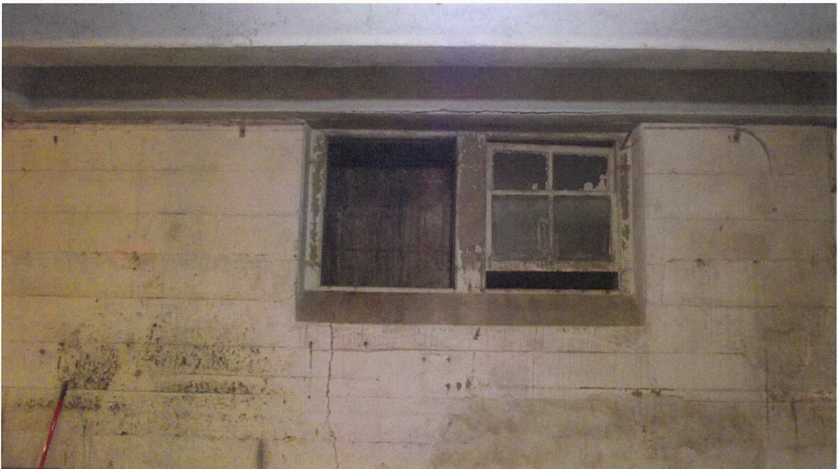
West inside view of basement
