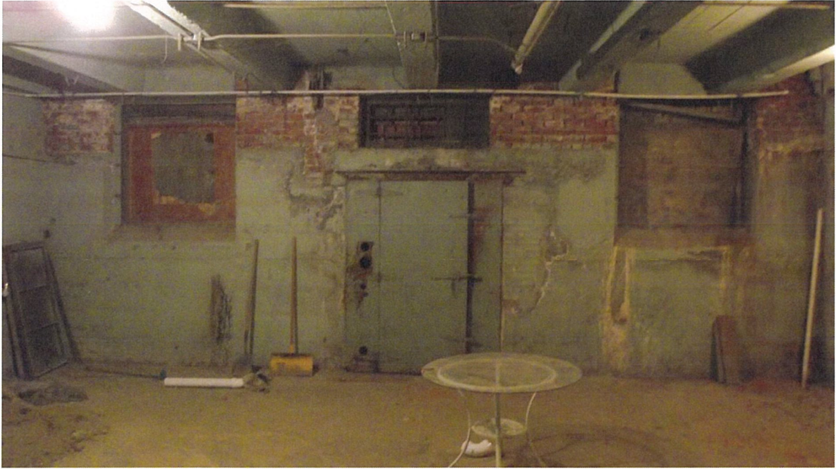
South inside view of basement
